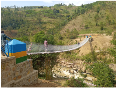
Figure 2: One of the over thousands trailbridges built by BBNP in Rwanda. This bridge connects Minazi and Mataba Sectors, spans 52 meters, and serves an estimated 2,860 individuals.
